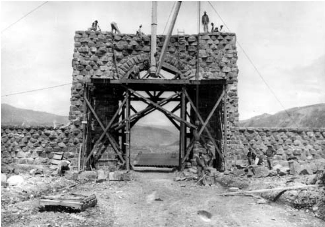
A rare photo of the arch under construction, summer 1903.
