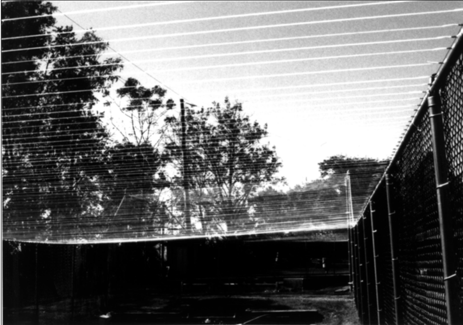
Figure 4 —Overhead wires can make a durable, all-weather exclusion system. Attaching such a system to a tall fence makes
