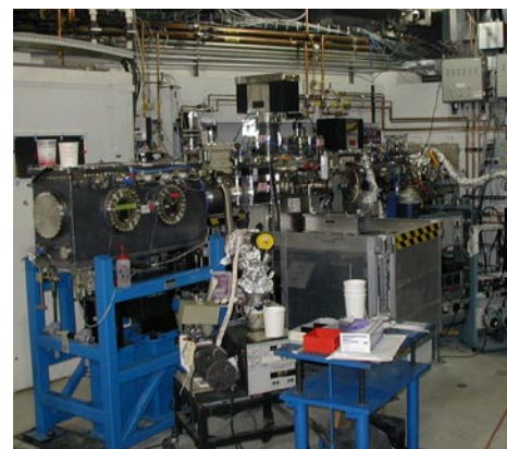
The 'new' X3 beamline under construction during the Spring 2006 shutdown.
