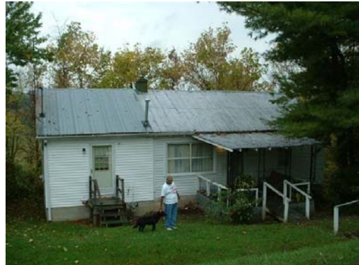
William and his dog, before repairs were made.
