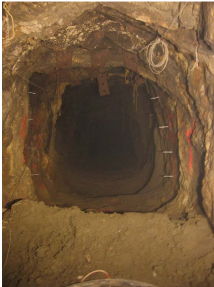
Figure 5. Army Tunnel conditions prior to bulkhead construction (future bulkhead location indicated by sidewall anchor bolts).
