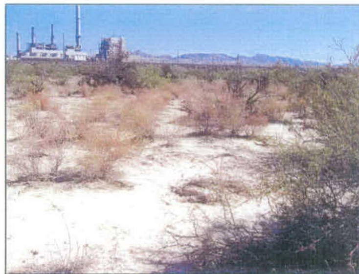
View looking southeast, showing Nevada Power Generating Station.
