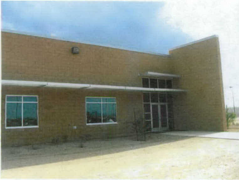
Typical Public/Staff Entrance
