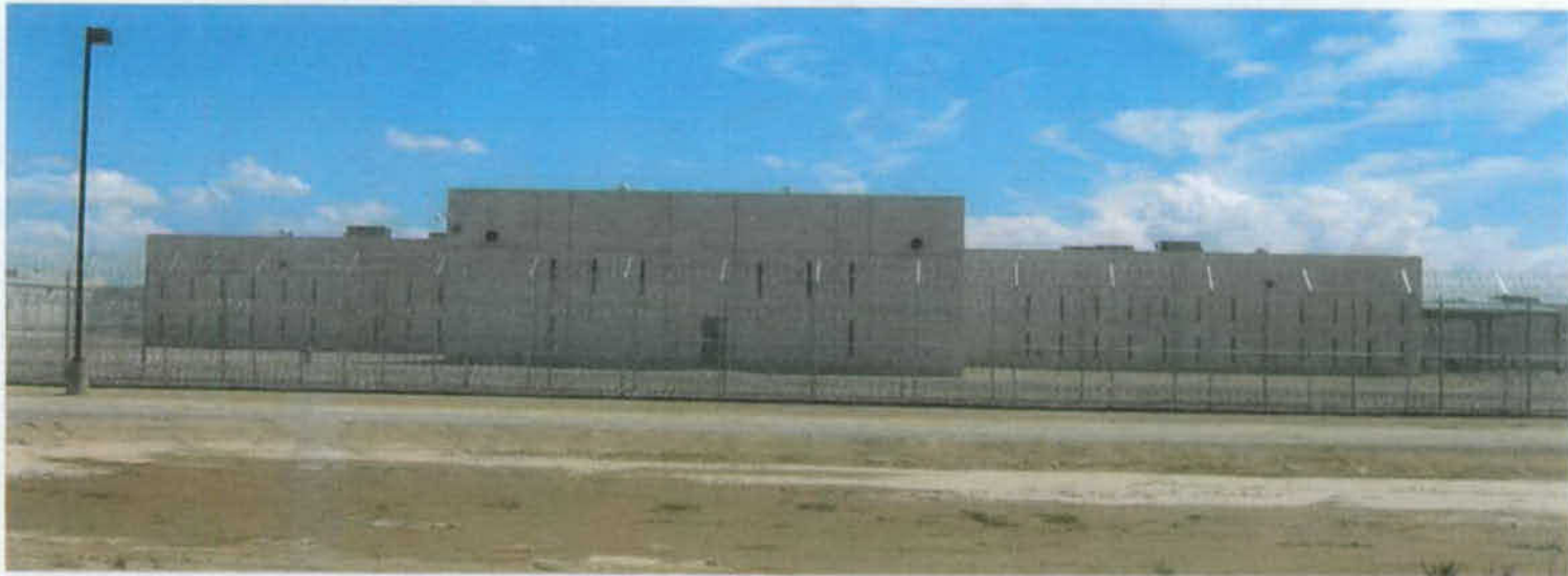
Typical Secure Housing, Perimeter Fence
