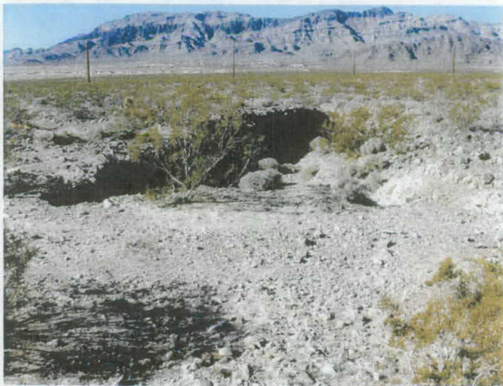
Photograph 14. View of the drainage feature at photo location 14, looking downstream.
