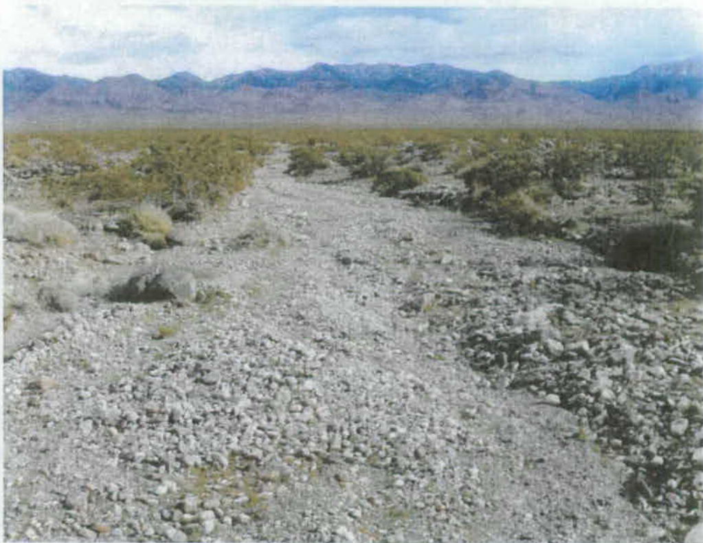
Photograph 6. View of the drainage feature at photo location 6, looking upstream.
