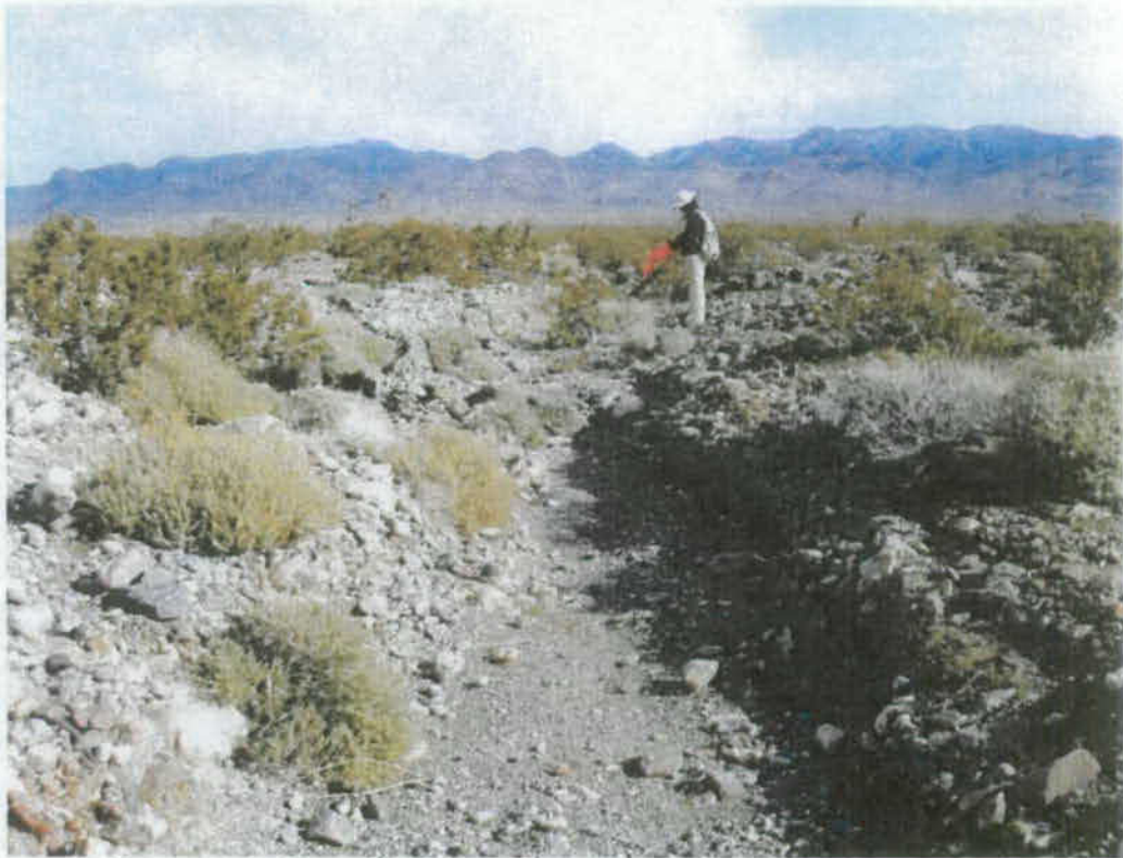
Photograph 2. View of the drainage feature at photo location 2, looking upstream.
