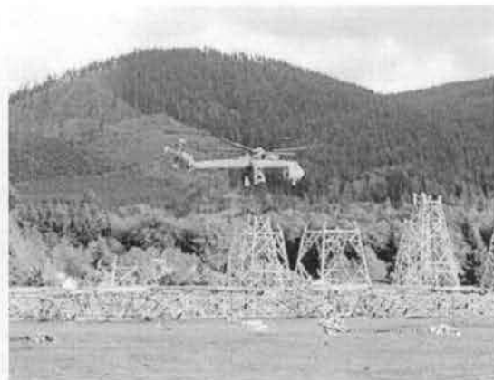
FIGURE 3.9-1 Towers under Construction
