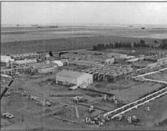
Typical natural gas compressor station
