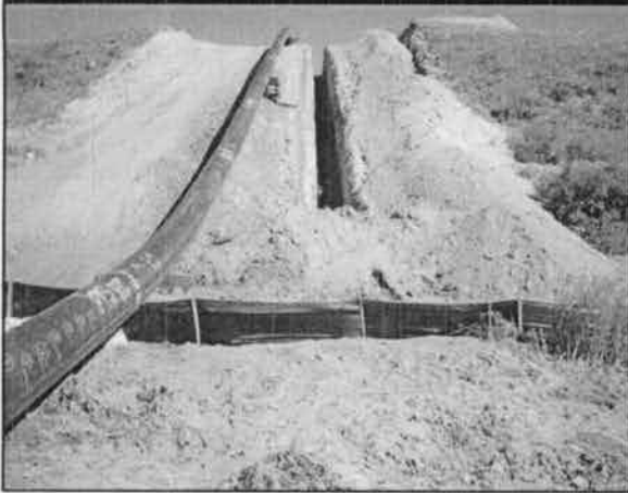
Trenching in preparation for installation of gas pipeline
