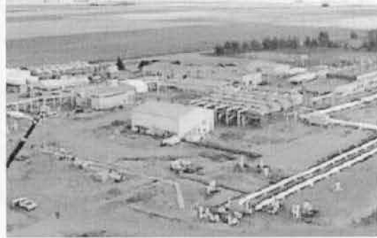
FIGURE 3.9-6 Typical Natural Gas Compressor Station
