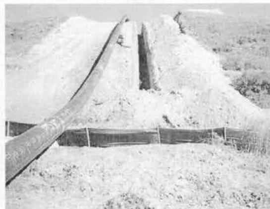
FIGURE 3.9-2 Trenching in Preparation for Installation of Gas Pipeline
