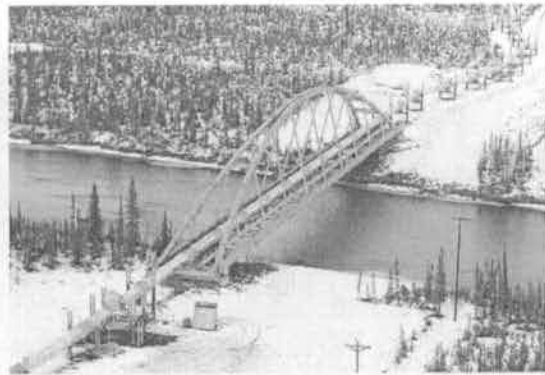
FIGURE 3.9-9 Trans-Alaska Pipeline Bridge over Gulkana River
