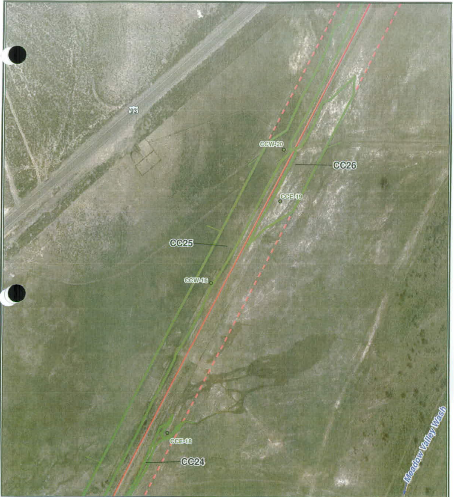
Figure 40 Caliente Rail Corridor Wetlands Caliente Segment
