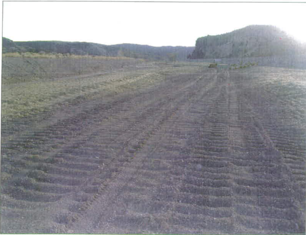
Photo 1. Photograph of WOUS 19D showing the re-shaped channel on Clover Creek.
