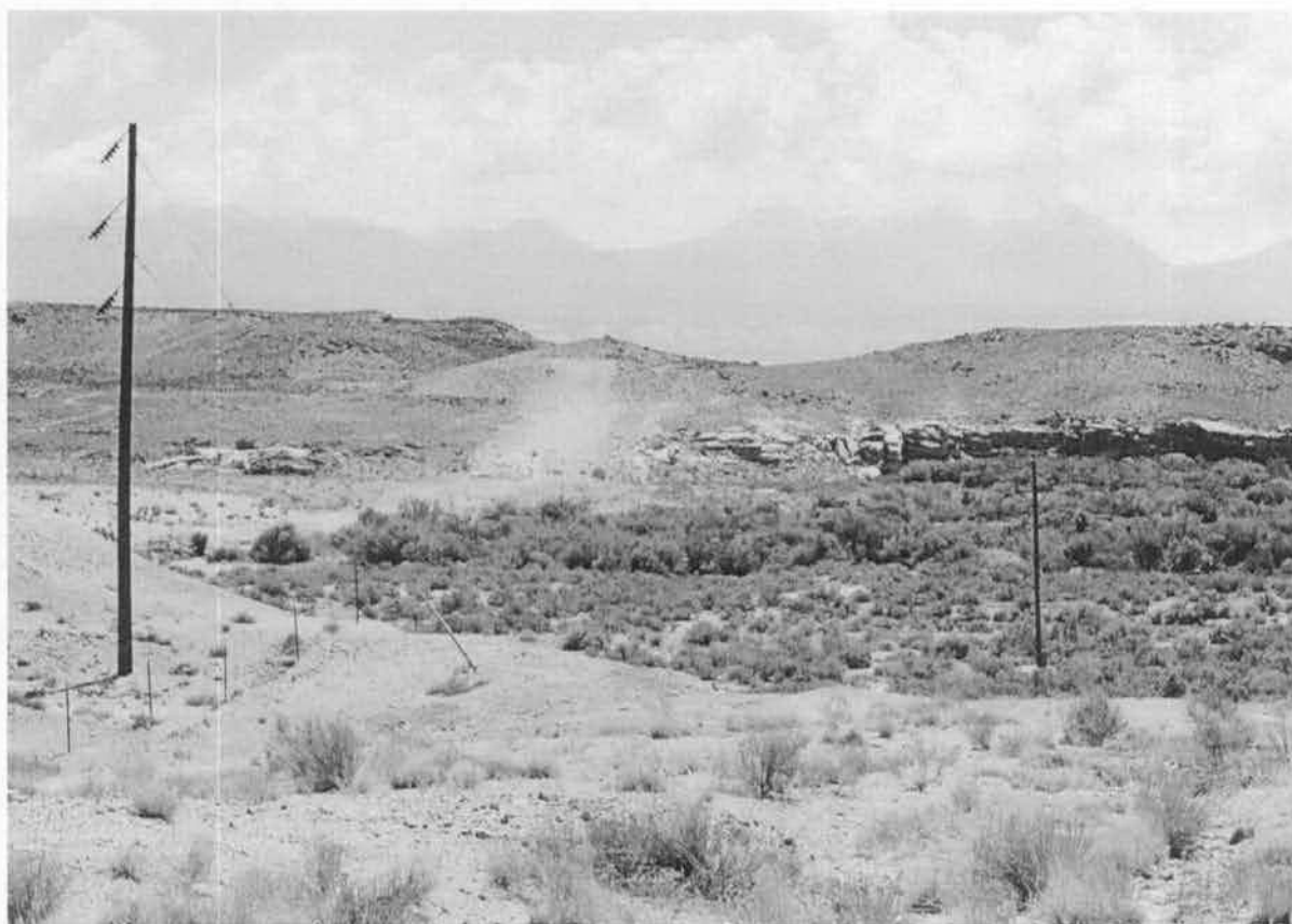
Figure 4-12. View of 5-Year-Old Pipeline Corridor from US-191, Approximately 2 Miles South of Blue Hills Road Turnoff
