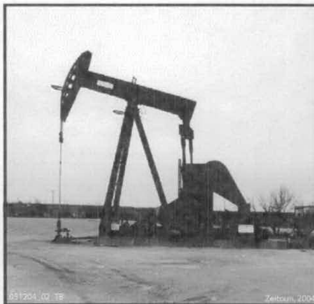
Figure 3-4 Oil Pump Jack
