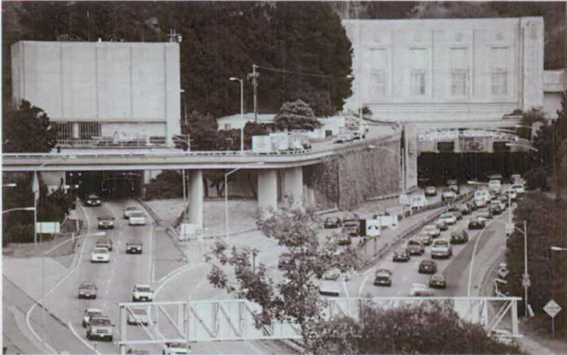
Figure 2.1. West Portal of Caldecott Tunnel
