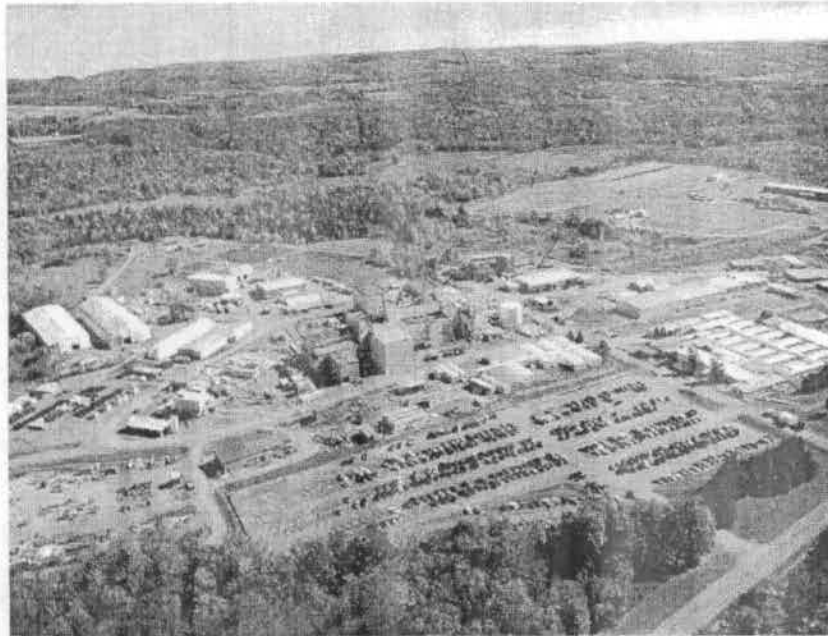
Figure 2-4. Aerial View of WVDP Site Facing Southeast
