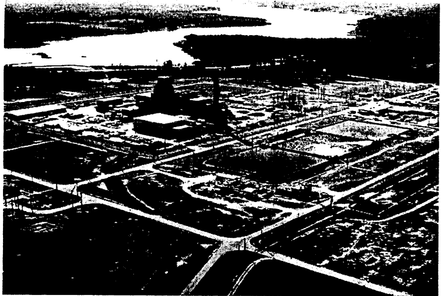
L-Reactor Complex at SRS
