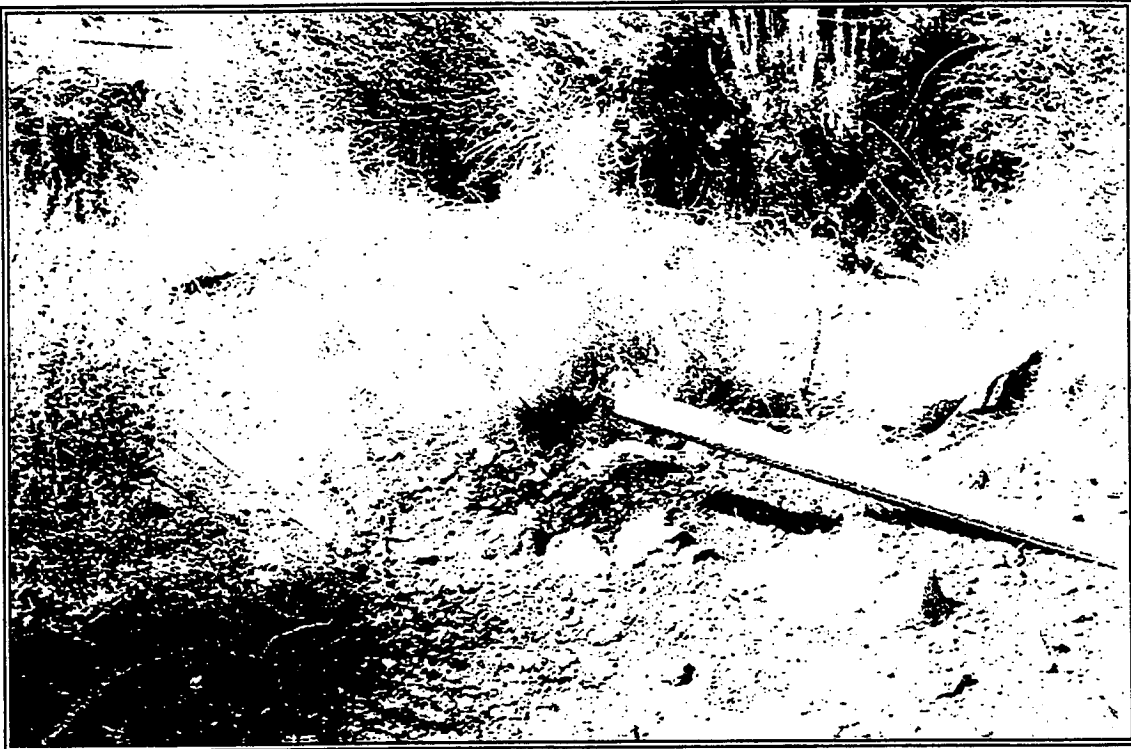
Photo 4-45 Outflow pipe at Topopah Spring on September 9, 1996 (WS340-10.TIF)
