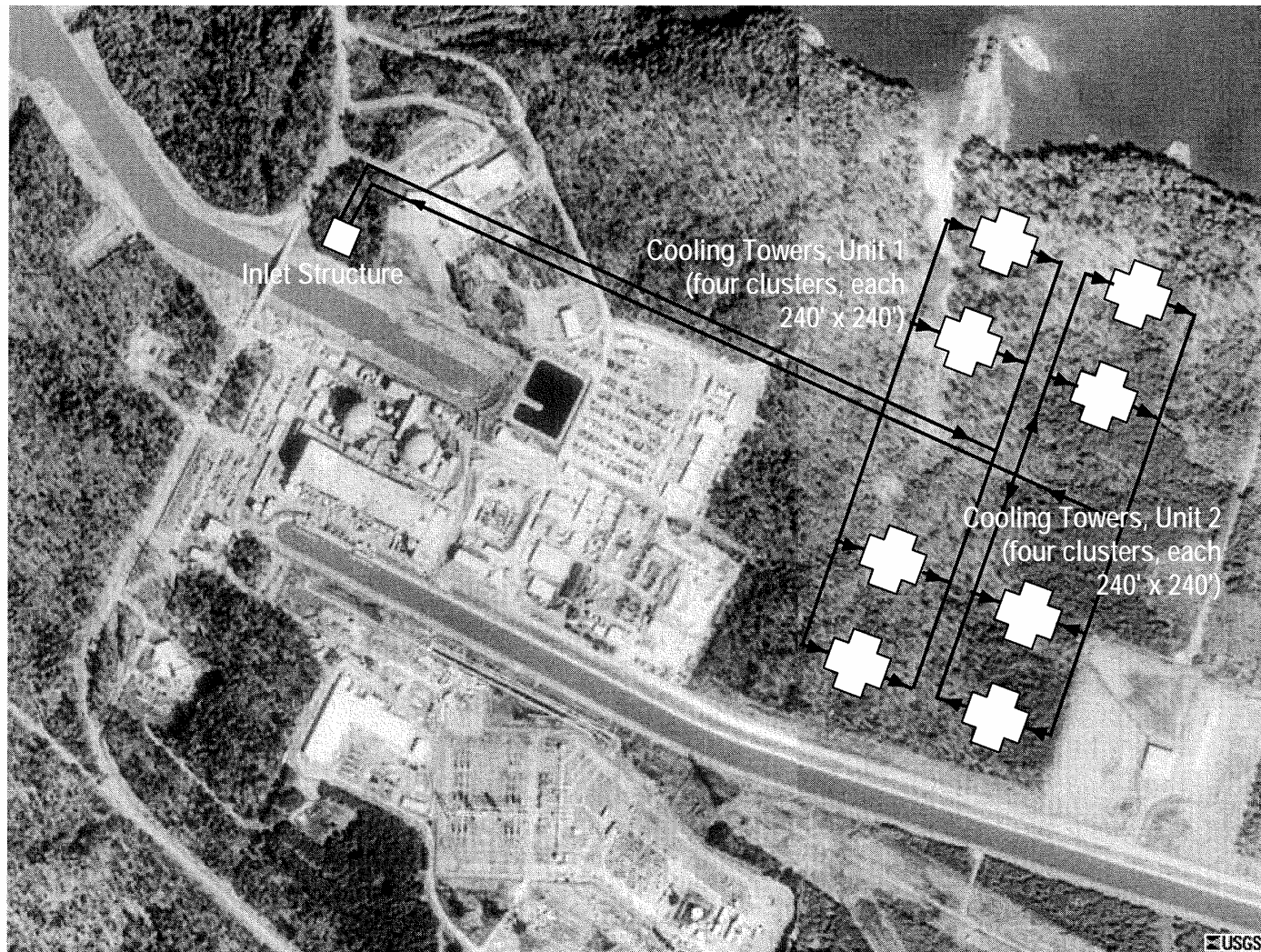
Figure 2-1 Aerial Photograph, Vicinity of Surry Site, with Proposed Cooling Towers Superimposed
