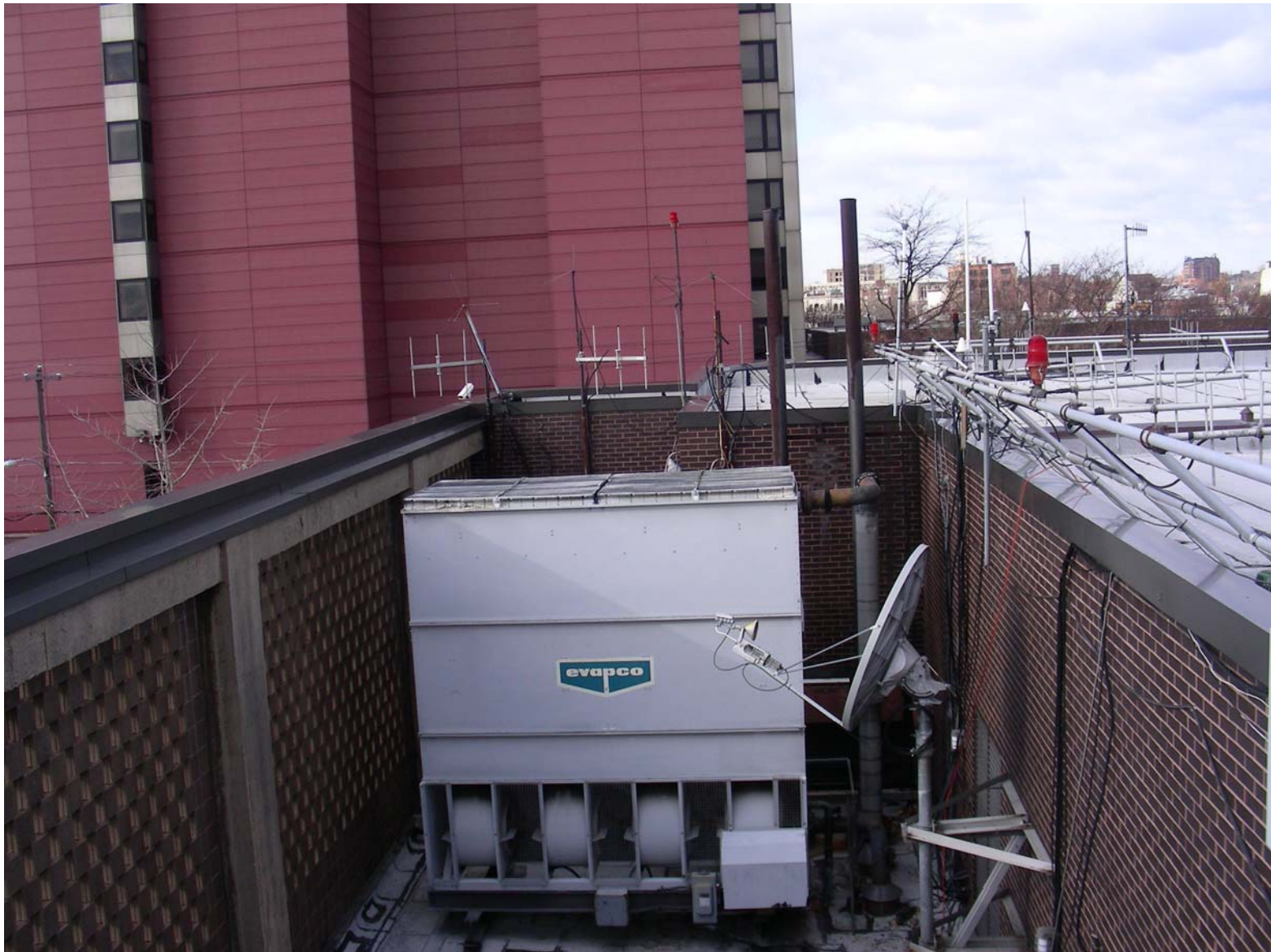
View of two emergency diesel exhausts and the mechanical area.
