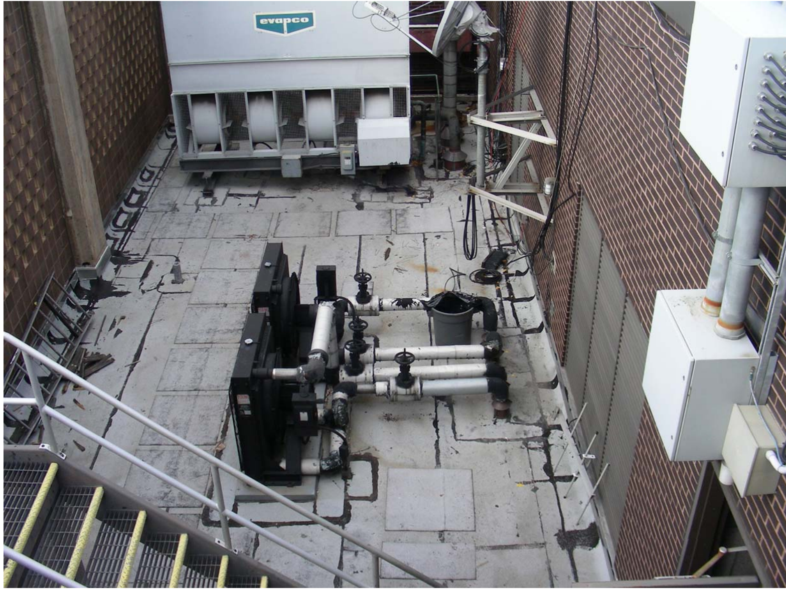
View of bottom of the mechanical area.
