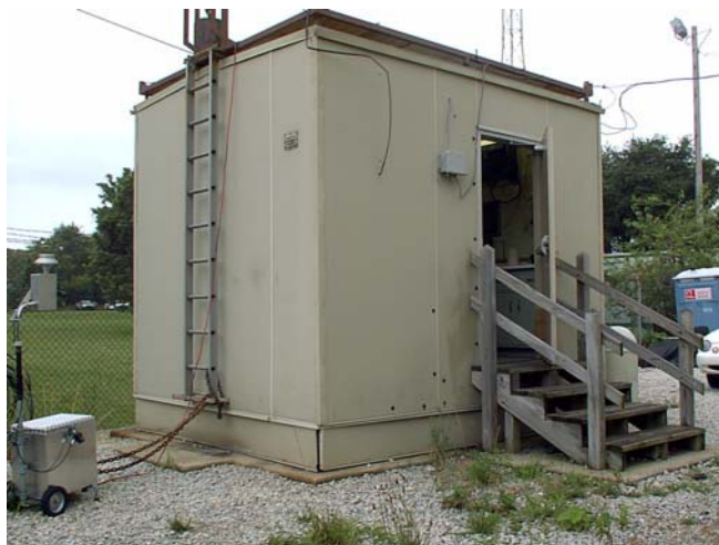
Figure 17 - Ground Level NEW Monitoring Station Picture
