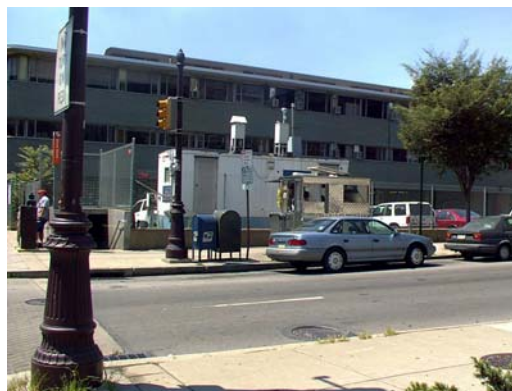
Figure 14 - Ground Level CHS Monitoring Station Picture
