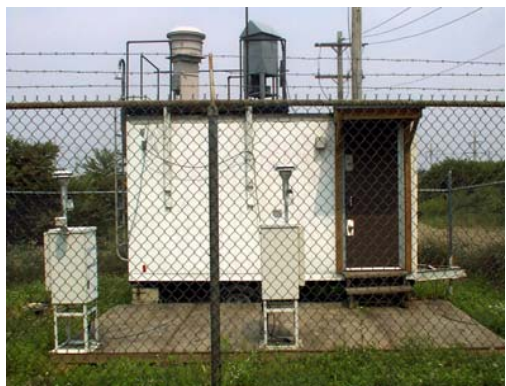
Figure 11 - Ground Level ELM Monitoring Station Picture
