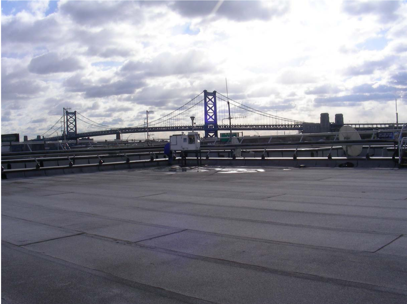
Fire Dept. HQ PM 2.5 Sampler on roof.
