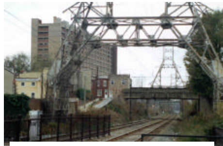
Public transportation near building to be imploded
