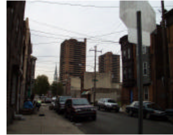
Homes near implosion site
