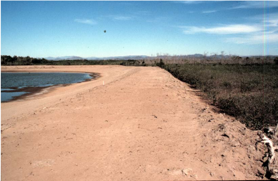
3-5. Example of a levee around a shrimp pond.
