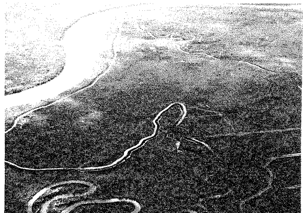
Figure 46. The extent of diking by agricultural interests along the western bank of the lower Apalachicola River.
