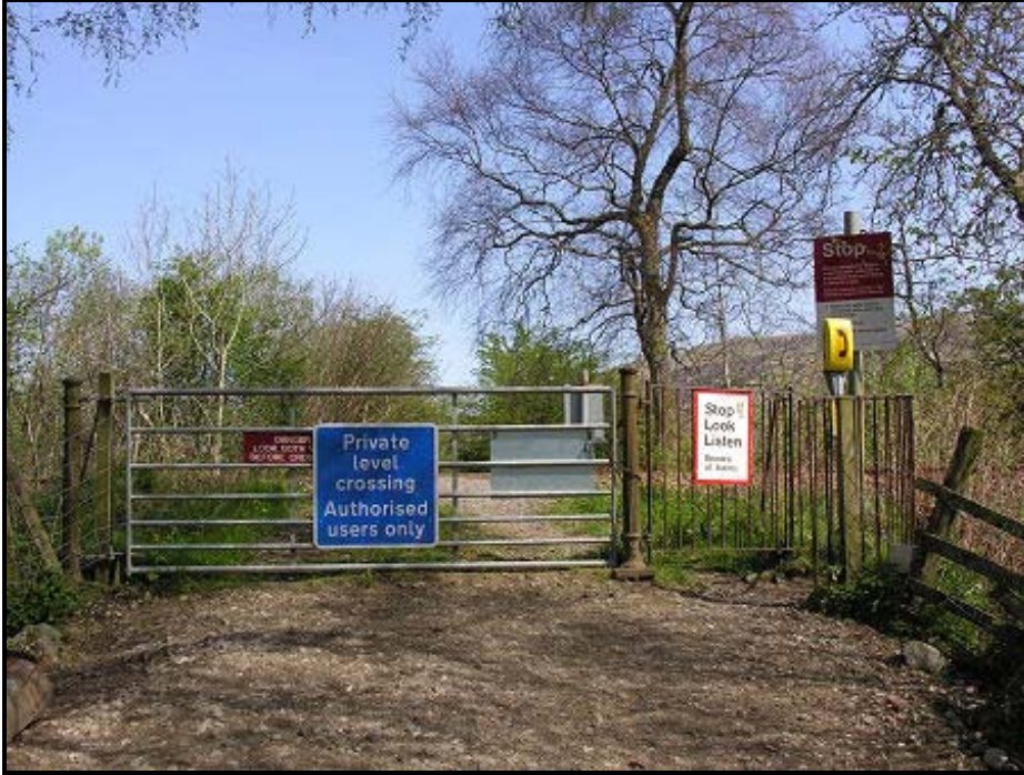
Figure 25. Private Highway-Rail Grade Crossing in Great Britain
