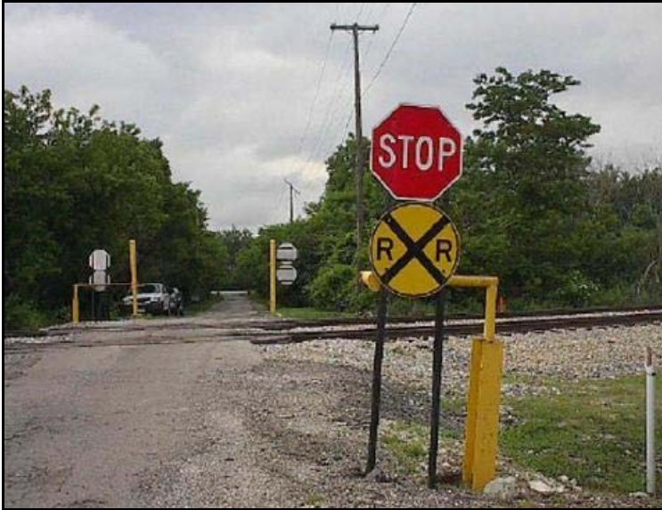
Figure 36. Additional Private Crossing Signage Example
