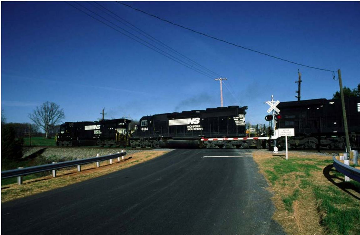
A set of three locomotives runs across a rural grade crossing equipped with flashing lights and gates, which are fully activated. The roadway has been recently paved, and a stop bar is visible at the crossing.
