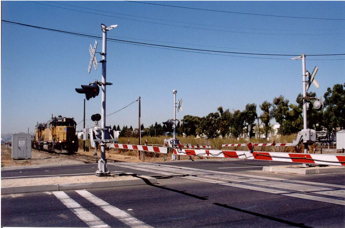
A four-lane divided highway at a grade crossing, with lights and gates fully activated. In the distance, a pair of freight locomotives can be seen moving toward the crossing.
