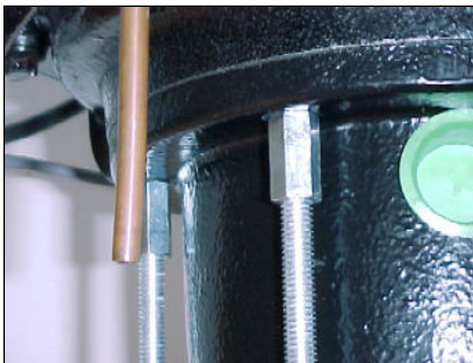
Figure 2: Close-up of installed allthreads.
