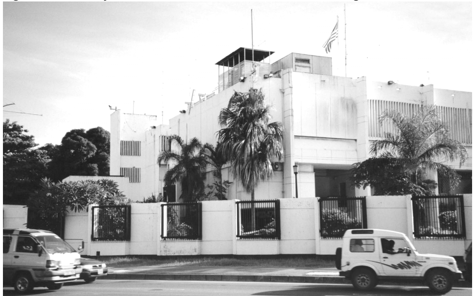
Figure 8: Embassy in Dar es Salaam, Tanzania, Before Bombing
