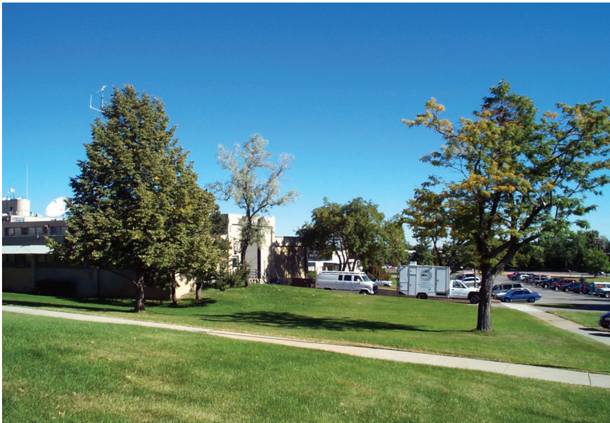
Department of Commerce Boulder Labs. Top: radar measurements at Table Mountain field site; bottom: ITS vehicles parked in the back of the main facilities at 325 Broadway (photographs by F.H. Sanders).
