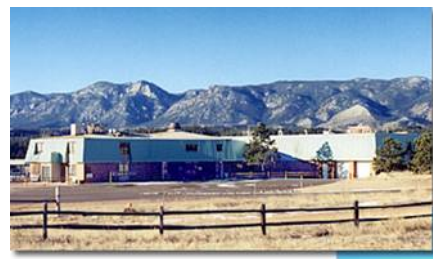
Figure 8 NAVSYS Building (Southwest View)
