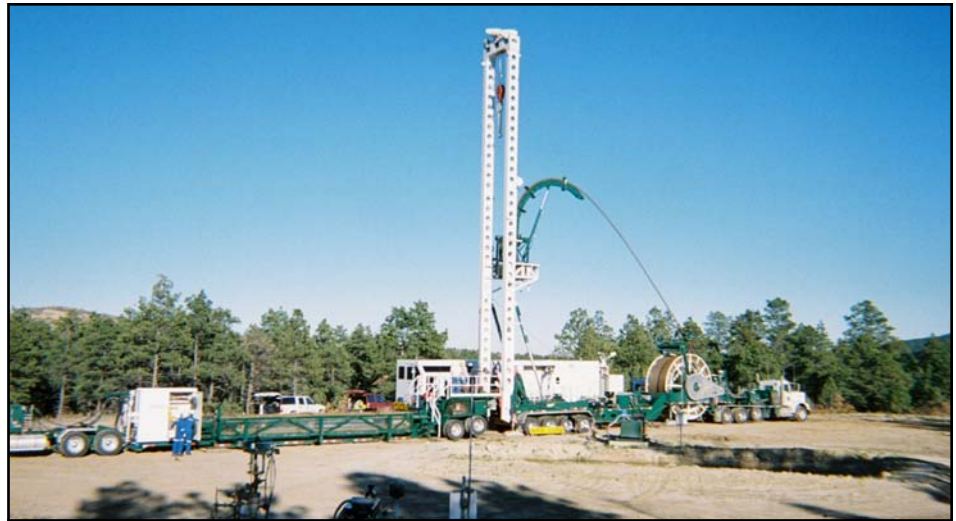
Coiled tubing unit to be modified.
