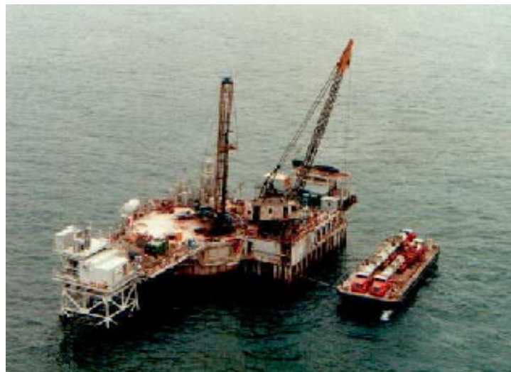
ExxonMobil's Belmont Island Removal Project
