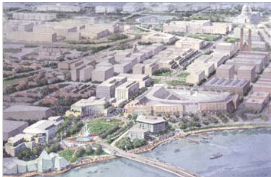
The new South Capitol Street corridor will feature not only the baseball stadium, but also new offices, residences, shops, and commemorative sites, as well as a waterfront park.
