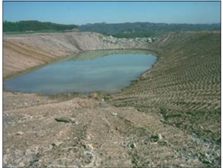
We ensure all surface water runoff from coal mines is routed through sedimentation ponds before leaving the permit area.
