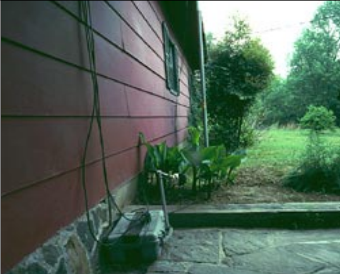
We monitor blasting to determine structural damage
