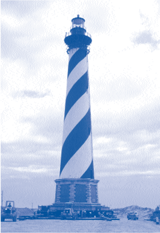
Cape Hatteras Lighthouse being moved from its original site.
