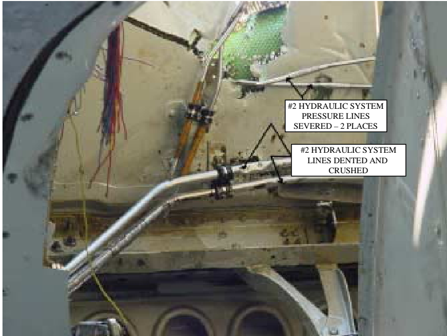
Figure 2 – Severed and Damaged #2 Hydraulic System Lines
