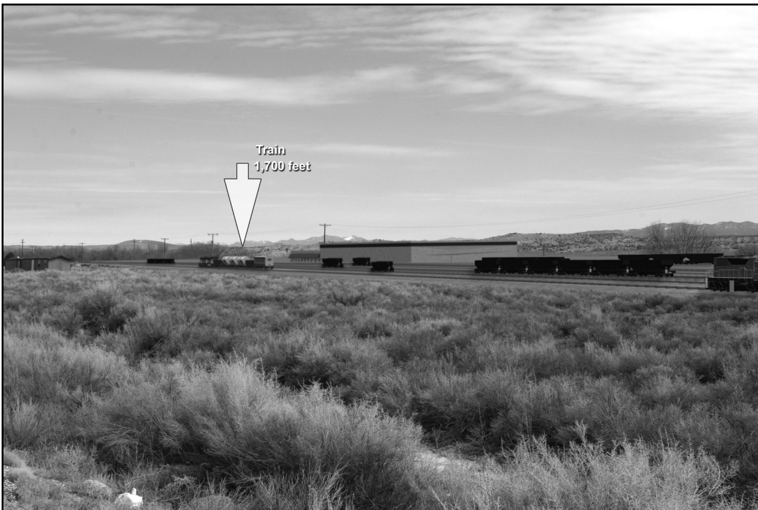
Figure D-11. Simulation of Staging Yard Caliente-Upland option in view north-northeast from key observation point 5.
