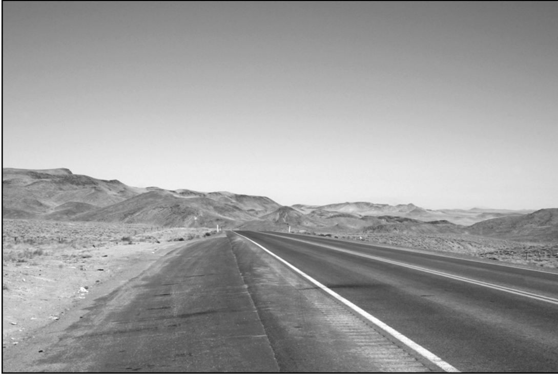
Figure D-91. View north in Long Valley, toward location of proposed grade-separated crossing of U.S. Highway 95 over Schurz alternative segment 5 from key observation point M-3.
