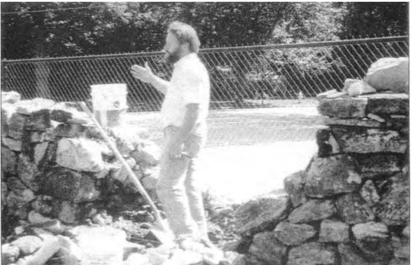
A section of a historic wall at Stan Hywet Hall in Akron, Ohio, was in need of restoration. Here, the limited replacement of a section of the wall was undertaken utilizing surviving stone and stones that matched the old in form, size, and color. Compatible substitute material could also have been used. (author, 1993)
