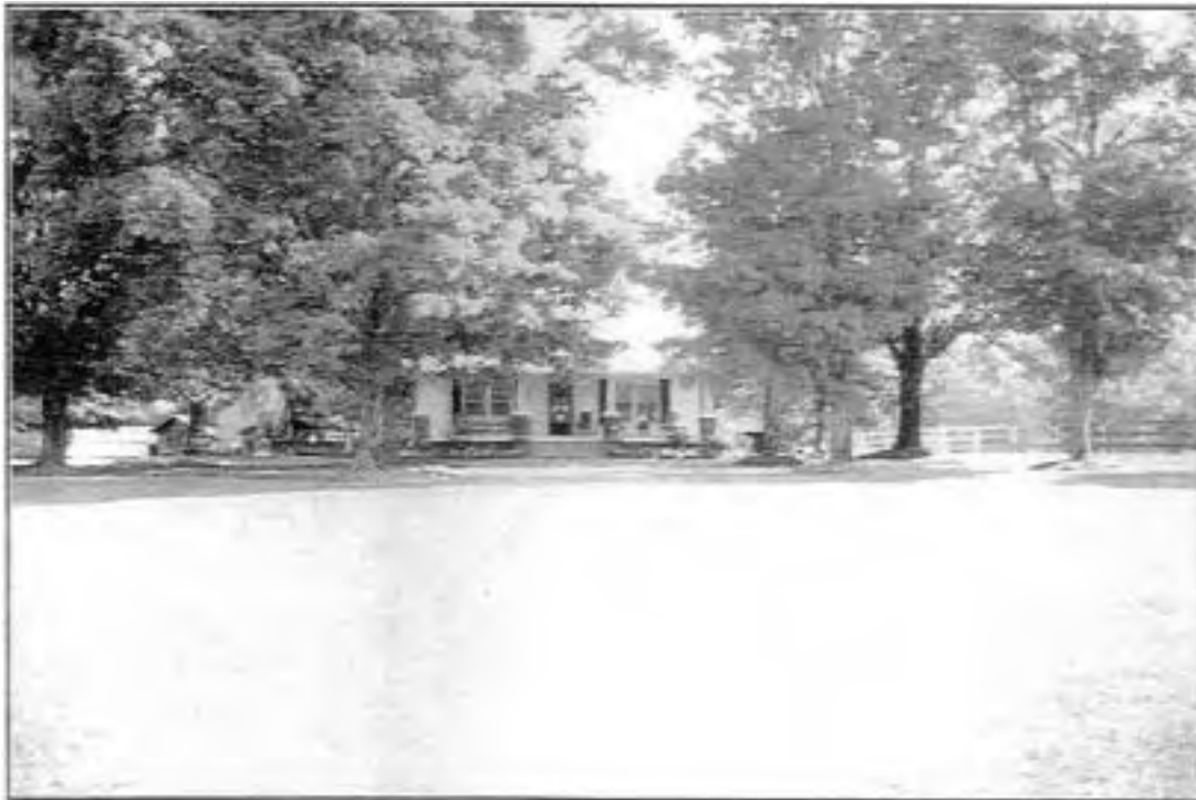
Neville Farm .View of agricultural complex of buildings, including bungalow residence
