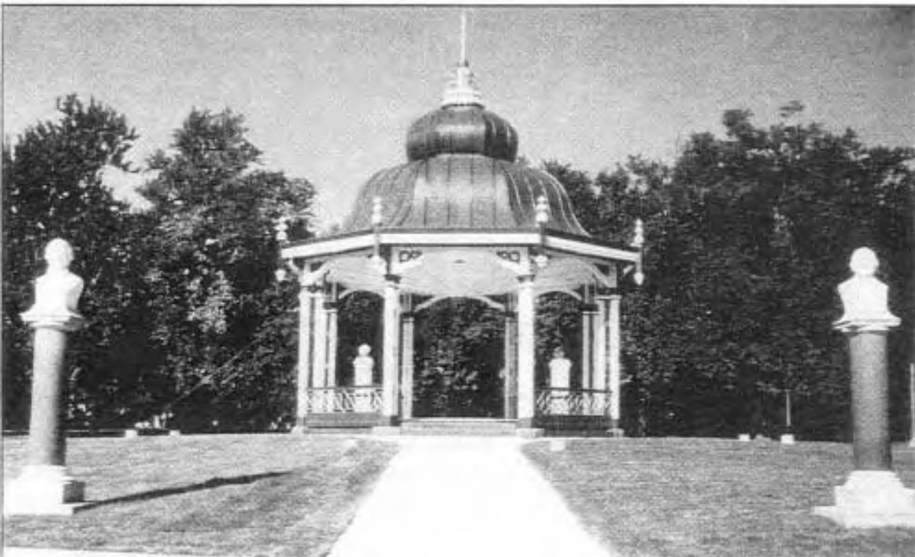
The area known as the music pavilion at Tower Grove Park in St. Louis, Missouri, had been badly deteriorated including its central marble busts, radiating walks, lawn areas and curbing. Utilizing photographic documentation, [top] the pavilion [opposite top right] and its associated landscape were restored to portray the pavilion as it would have appeared at a certain time. For example, the marble busts of eminent composers were replaced with pre-cast concrete replicas of the originals [bottom, foreground]. (Tower Grove Park)
