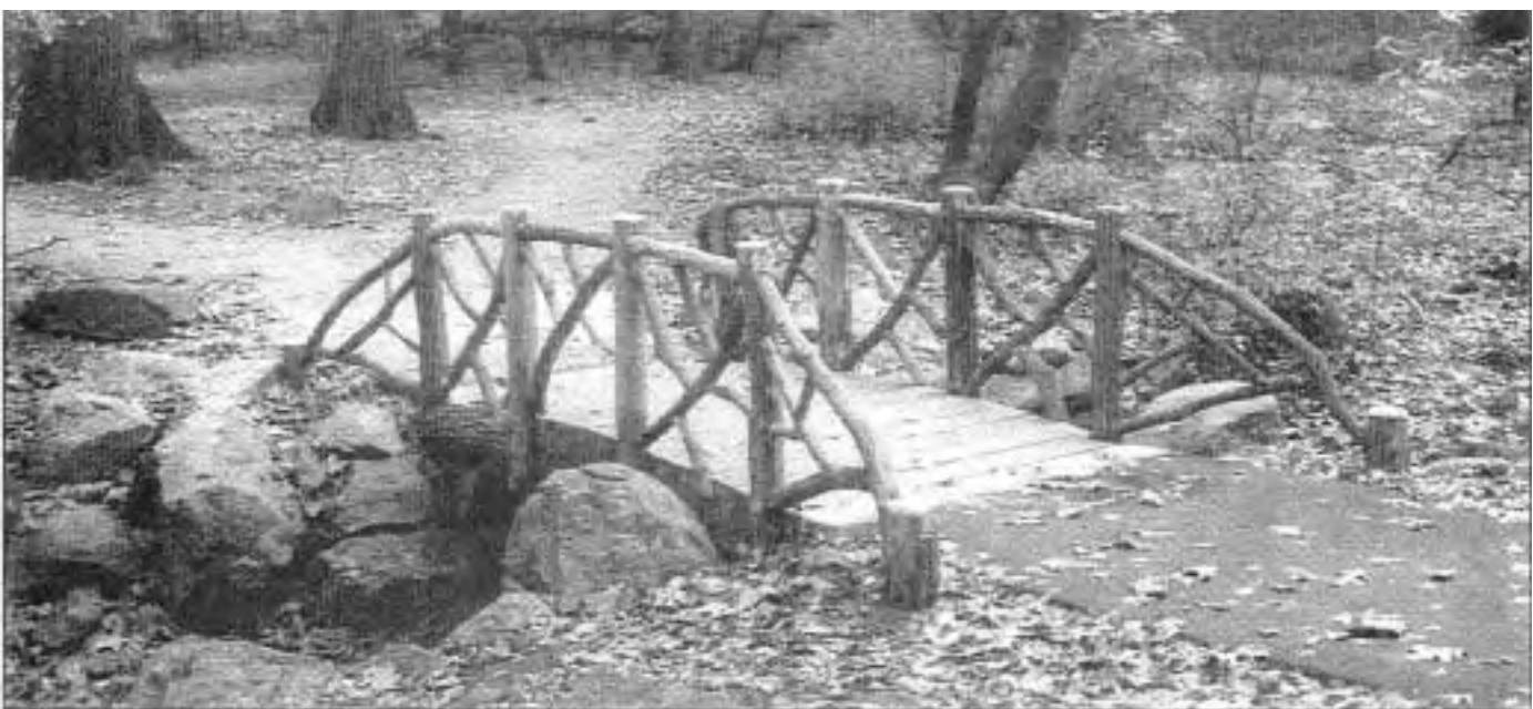
This small footbridge in Central Park's Ramble [above] has been re-created on the basis of historic documentation. The new bridge meets current code requirements, yet replicates the historic appearance, while utilizing compatible substitute materials. (Central Park Conservancy) The selected treatment for the landscape at the J. L. Bush Storehouse Property, Greenwich, Connecticut, [top] is restoration to the impressionist painters' period. Here, sensitive grading preserved historic landscape features while providing access on the alignment of the original path. For example, grade relationships to the historic building and hedge have been retained. (LANDSCAPES)
