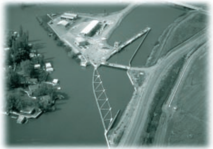
Tracy pumping plant and fish facility (photo by Reclamation).
