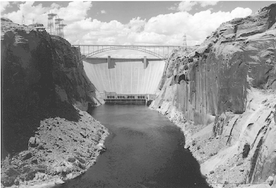
Looking upstream at Glen Canyon Dam and Powerplant.
