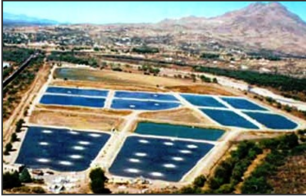
Nogales International Wastewater Treatment Plant
