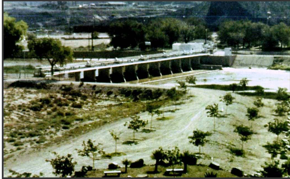
American Diversion Dam and Canal
