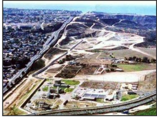
South Bay Int'l Wastewater Treatment Plant
