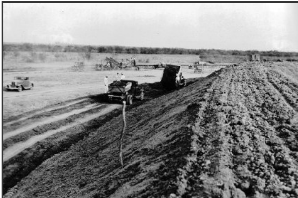
Lower Rio Grande U.S. Main Floodway
