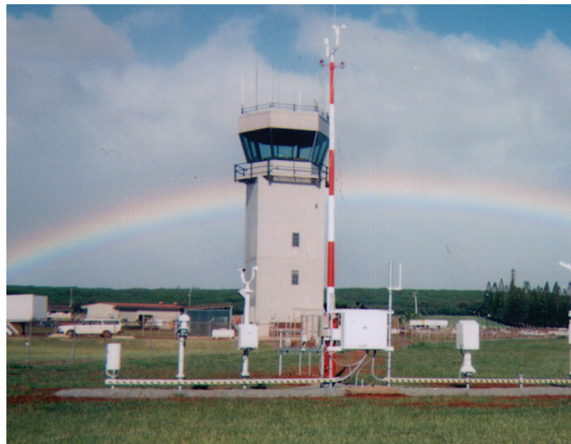
▲ ASOS installed near an airport tower.
