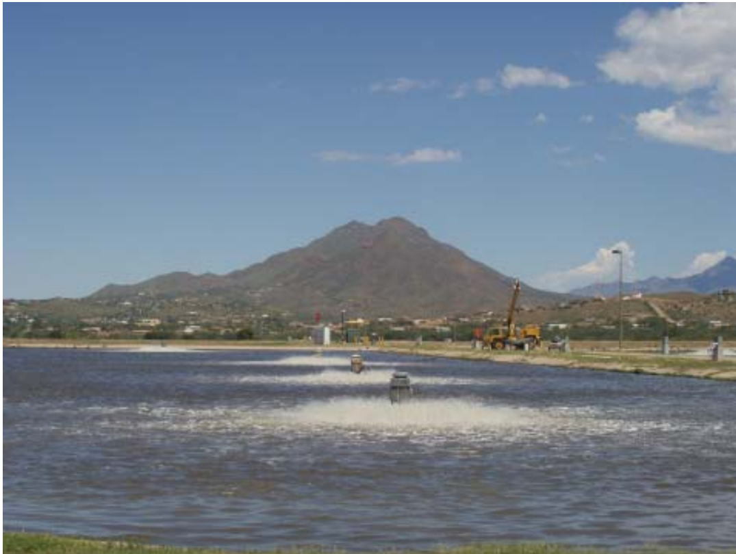
Nogales International Wastewater Treatment Plant
