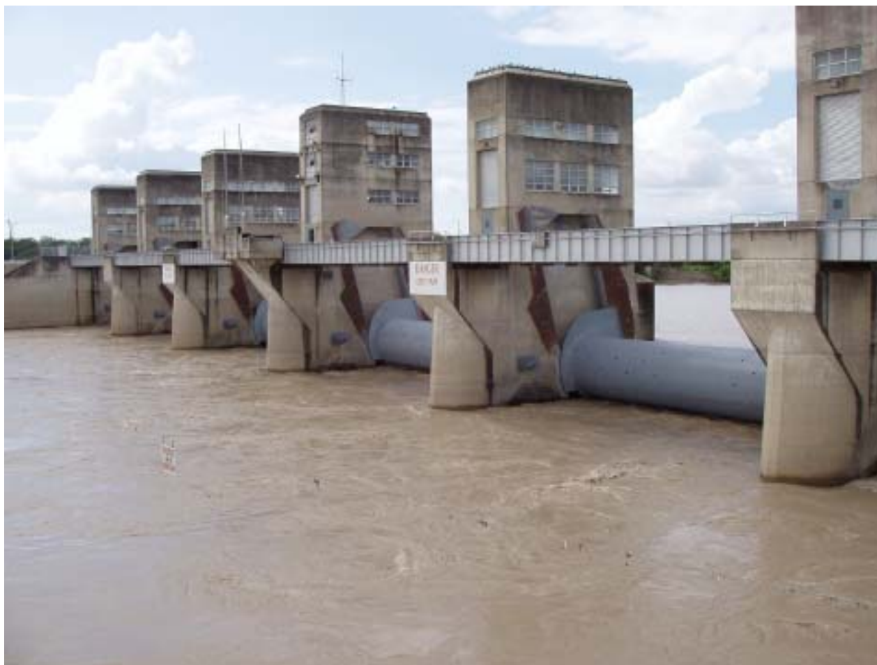
Anzalduas Dam during high flow
