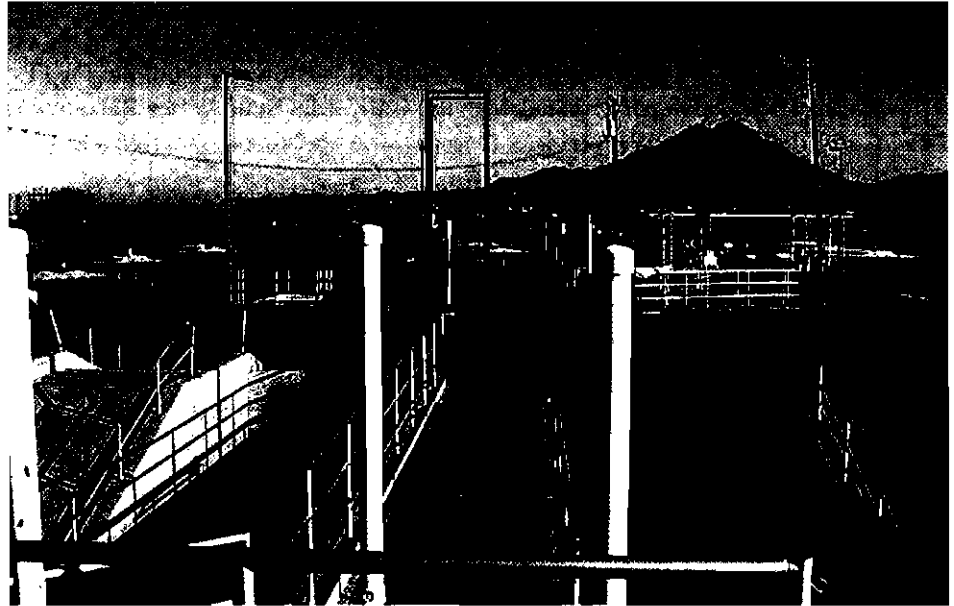
Nogales International Wastewater Treatment Plant
