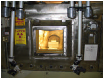
Hotbox facility (interior) with shielding to examine the irradiated fuel
