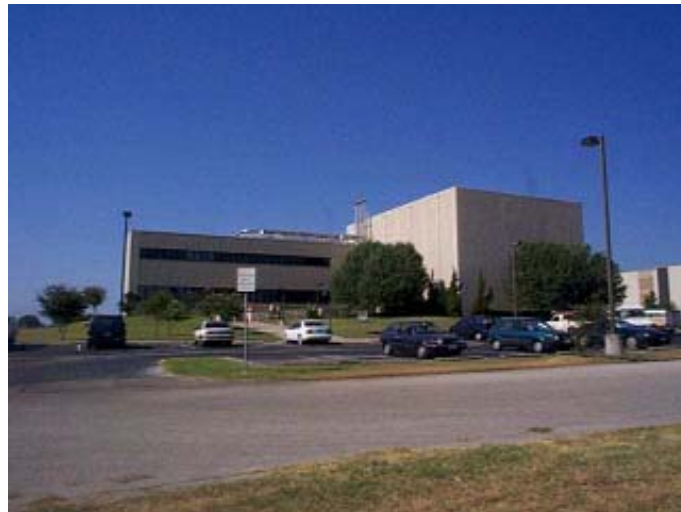
Nuclear Engineering Teaching Laboratory Building
