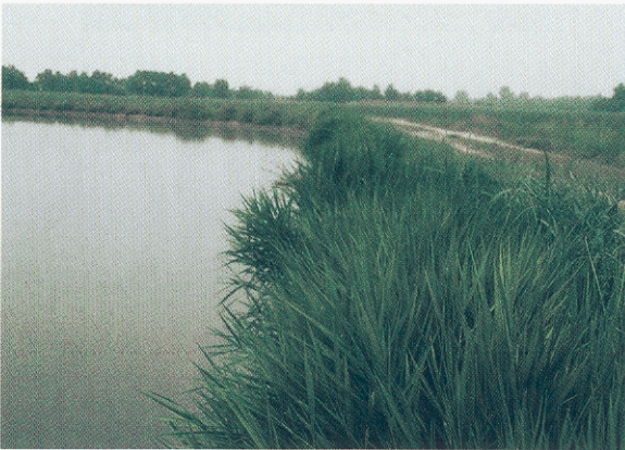
Controlling erosion along catfishpond levees
