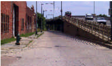
Existing Frederick Douglass Bridge ramp
