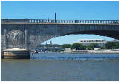
Memorial Bridge, Washington D.C.
