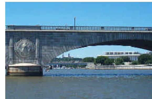
Memorial Bridge, Washington D. C.
