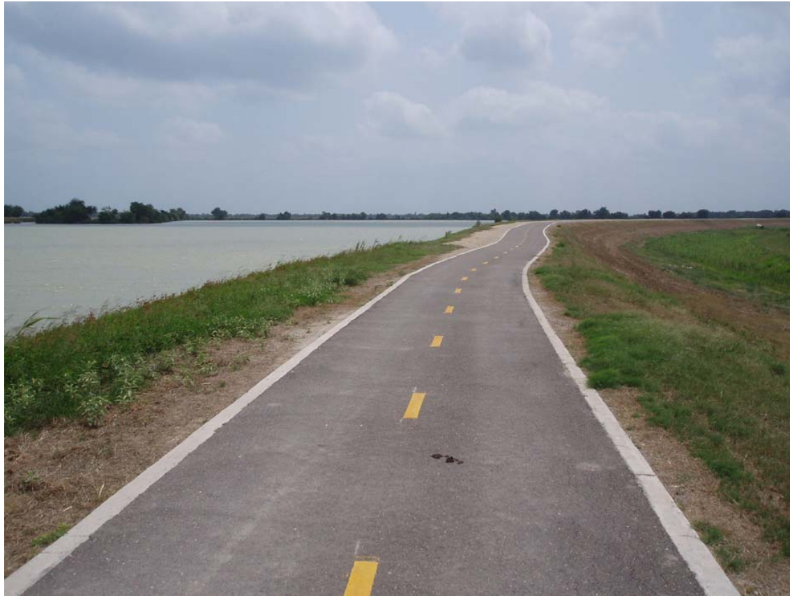
Levee was raised as part of the Hidalgo Hike & Bike Trail
