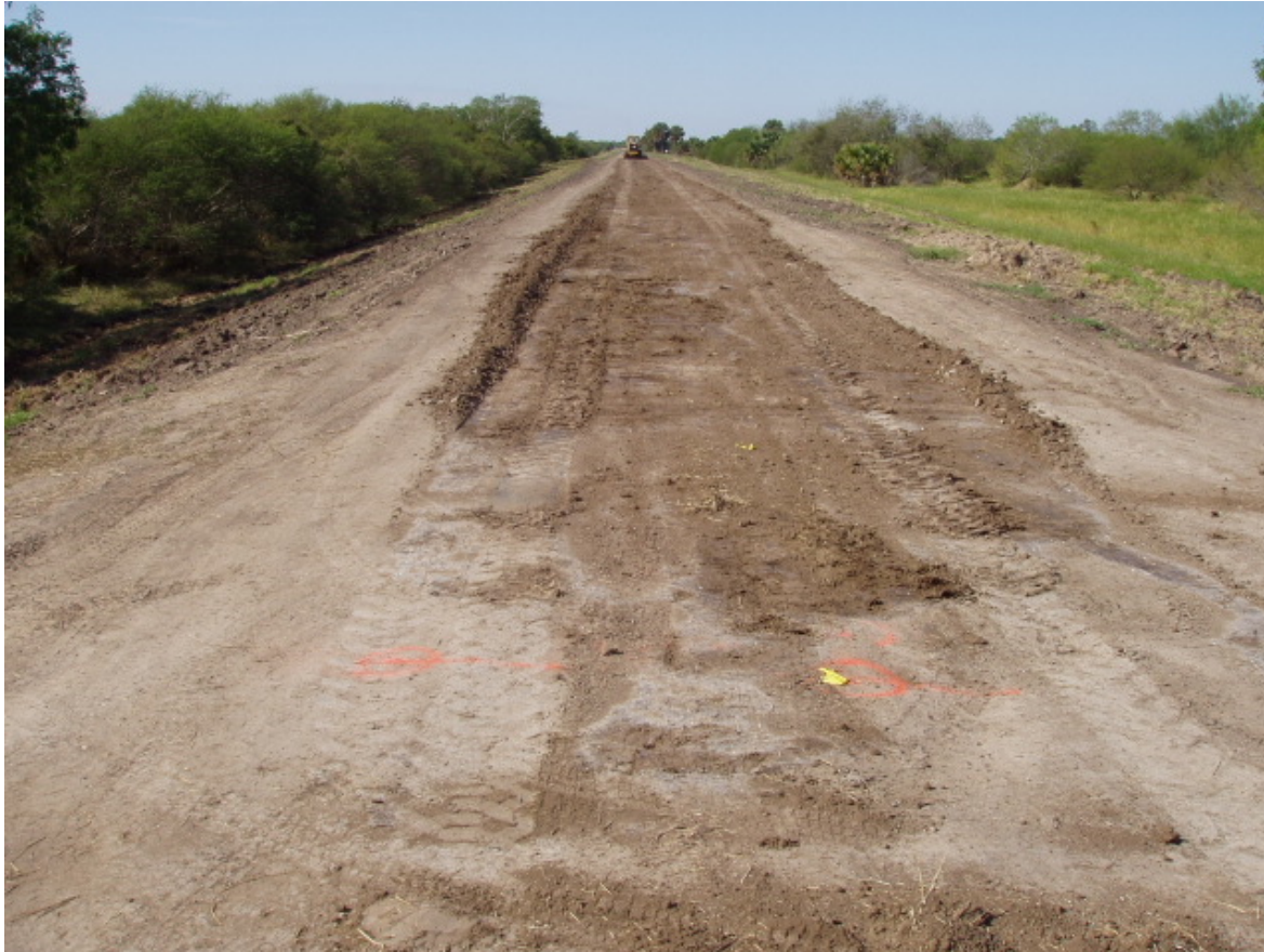
Preparatory work on levee near Sabal Palm
