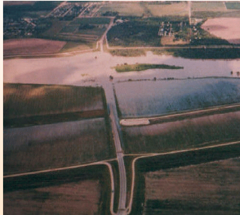
1978 Flood Divisor Dike with 10,000 cfs
