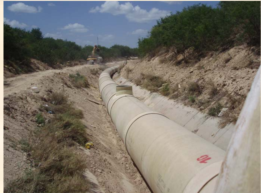
Connecting Pipe Sections
