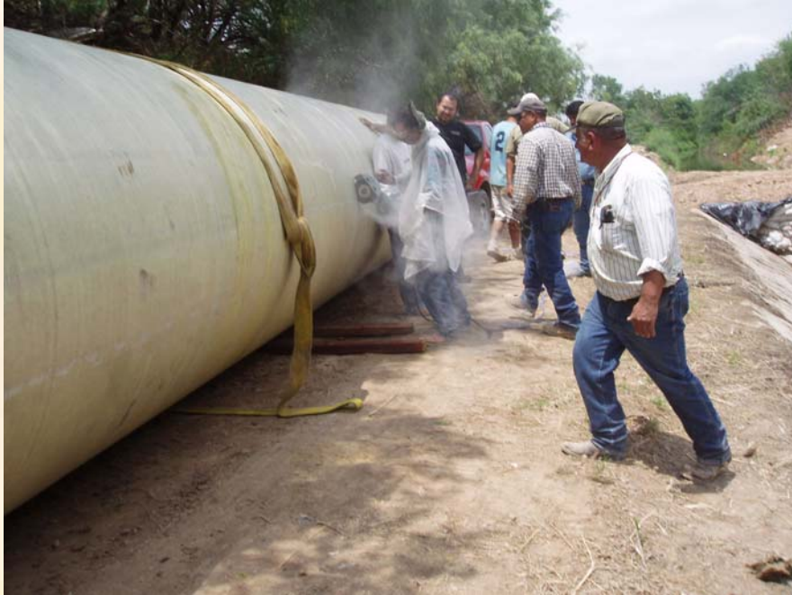
Cutting of Pipe Sections
