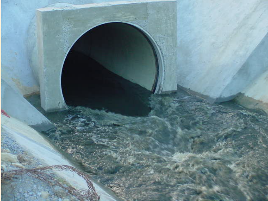
Water Discharged at Outlet Headwall
