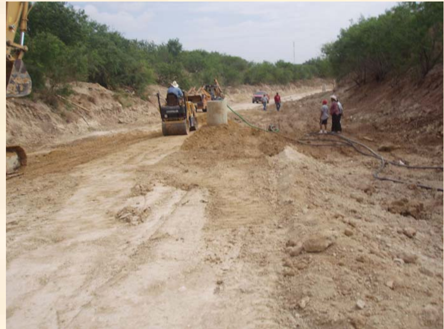
Compaction of Material Above the Pipe
