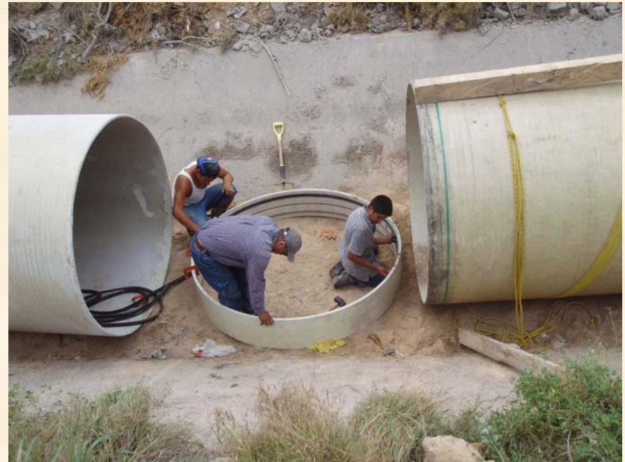
Installation of Seals at Pipe Joint
