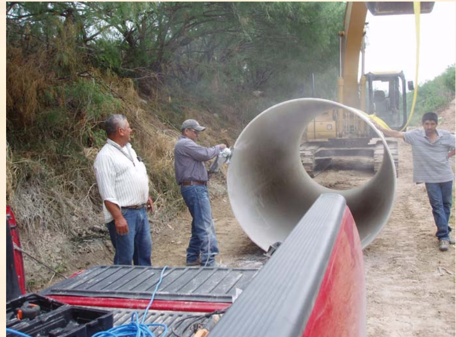
Preparation of Pipe Section before Installation
