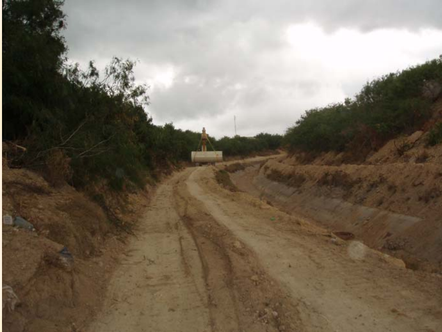
Hauling of Pipe Section by the Excavator
