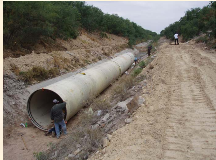
Laying of Pipe
