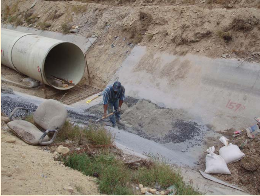
Start of Project – Pipe Outlet
