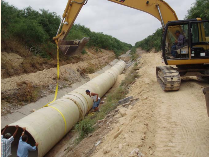
Connecting Pipe Sections
