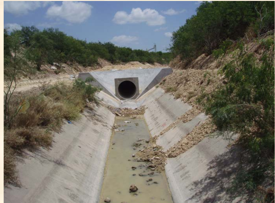
Finished Outlet Headwall
