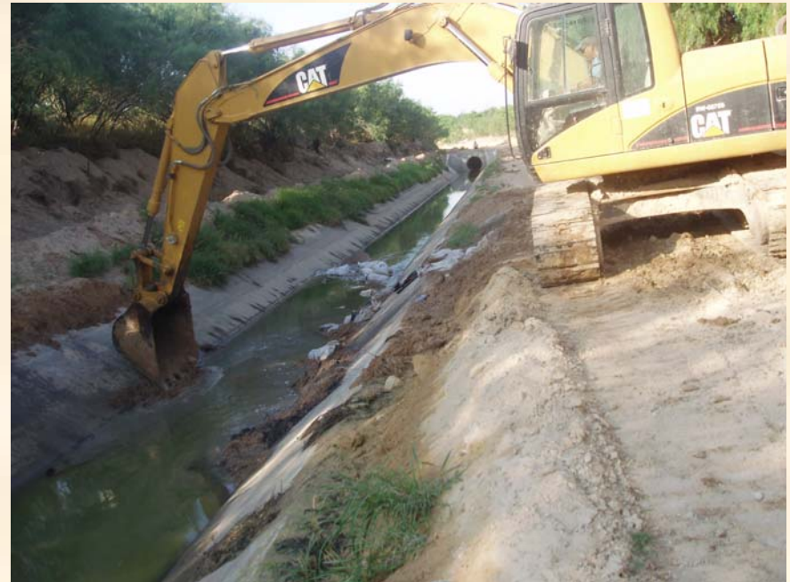
Removal of Berm in Canal
