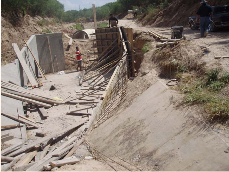
Construction of Inlet Headwall
