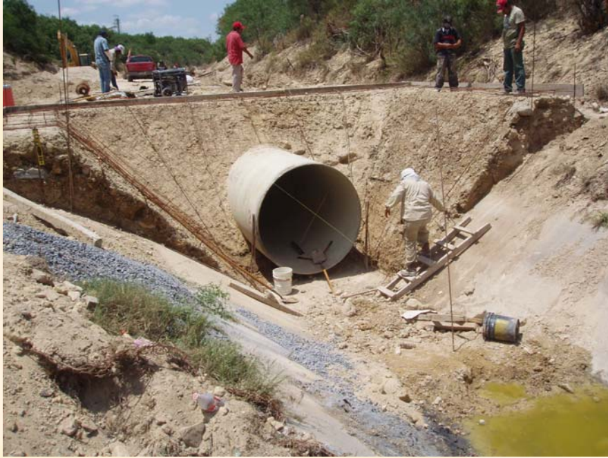
Construction of Outlet Headwall
