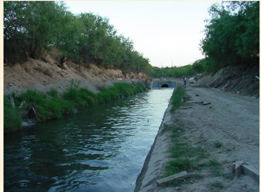
View of Canal and Inlet Headwall
