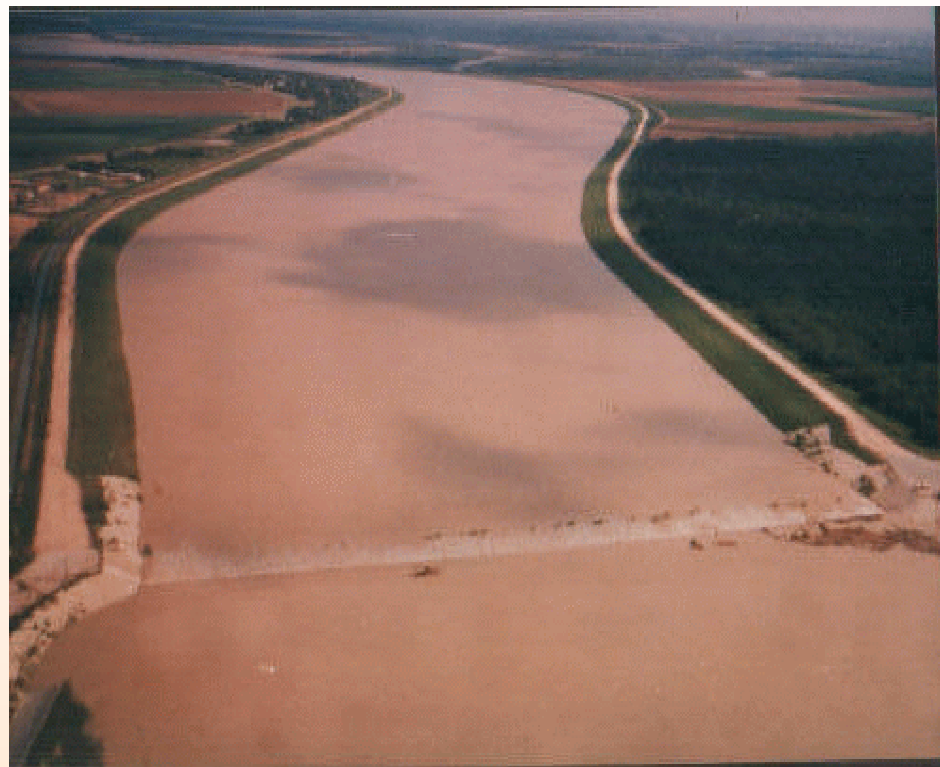
1978 Flood Banker Weir with 9,200 cfs
