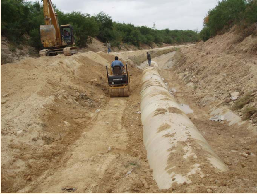
Compaction of Material Along Pipe
