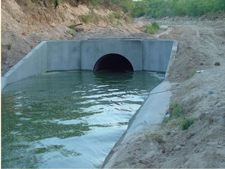
Water Released Into Inlet Headwall
