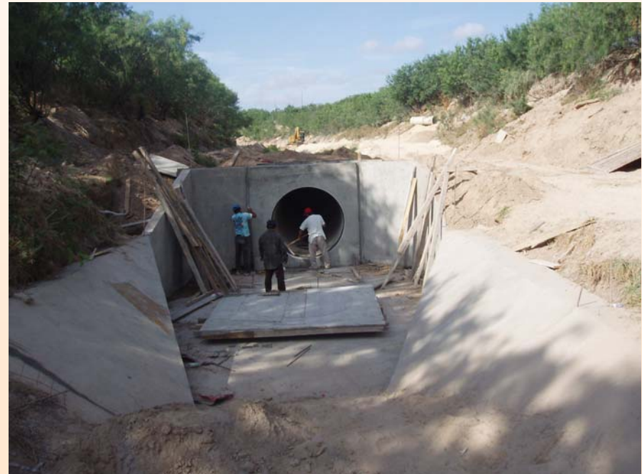
Finished Inlet Headwall
