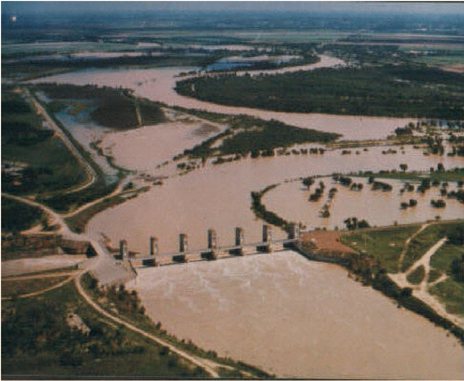
1973 Flood Anzalduas Dam
