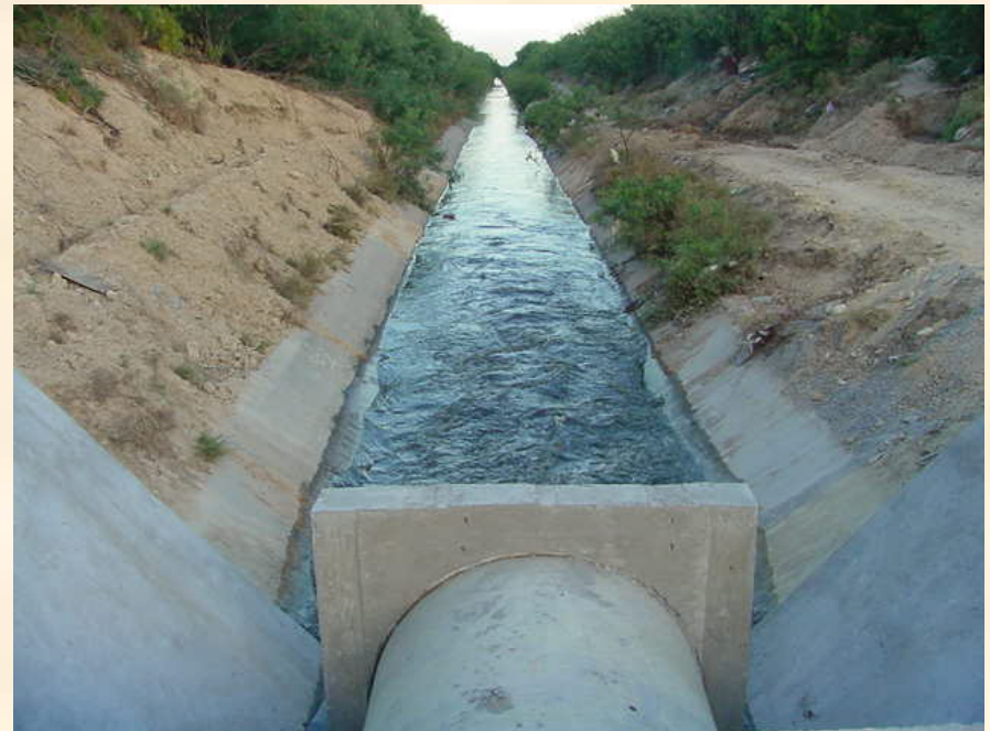
Downstream View of Canal
