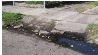
The Lodi Community Improvement Project aims to improve the infrastructure in most of Lodi east of Sacramento Street.
