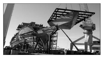
Rosslyn, VA – Jan. 26, 2006 – The final unit of the first Deepwater National Security Cutter (NSC), USCGC BERTHOLF (WMSL 750), was lifted onto the keel yesterday marking a significant construction milestone for the flag ship of the newest class of Coast Guard cutters. The first of eight NSCs being built by Northrop Grumman Ship Systems under contract to Integrated Coast Guard Systems (ICGS) has all assemblies on keel and is one step closer to reality.
