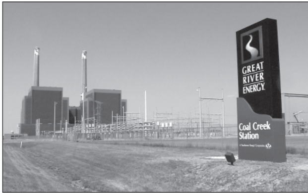
Great River Energy's Coal Creek Station, Underwood, North Dakota
