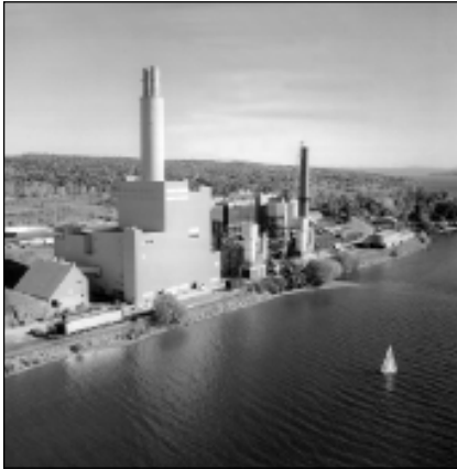
Milliken CCT project, with S-H-U scrubber in foreground.
